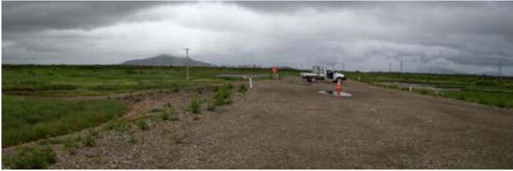
Fig. 5 Completed GTP on Townsville Port Access Road Project
