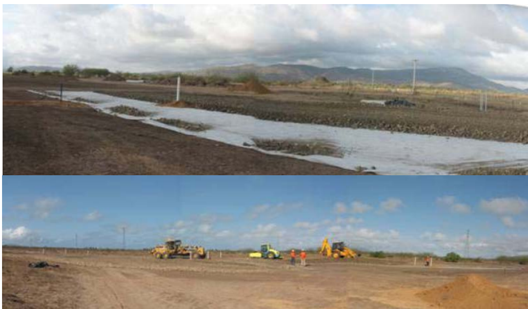
Fig. 4 Installation of Instrumentation and Construction Activities for GTP
