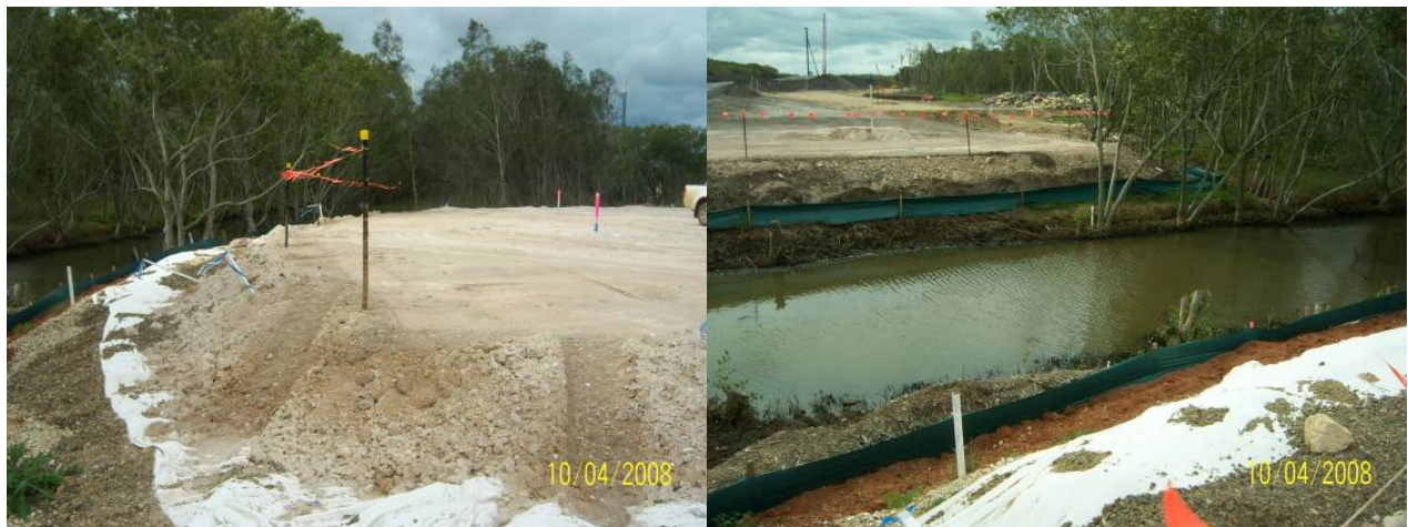
Figure 7. Polyfelt WX installed at BR25A and BR25B
